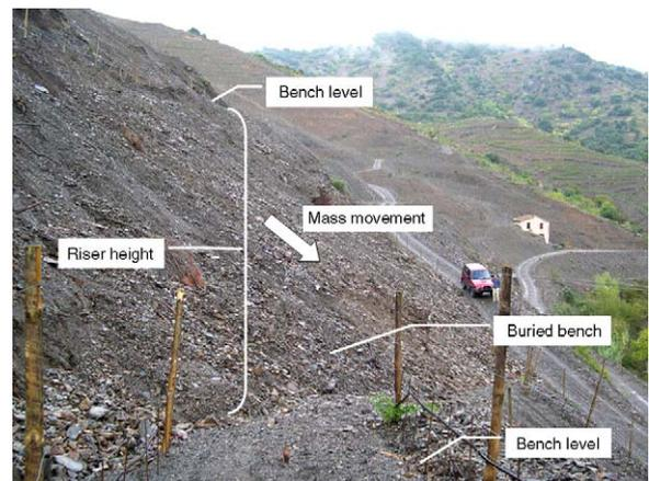
Fig. 6. Mass movement produced by the collapse of a riser in an area with excessive filling of materials and high slope degree.
