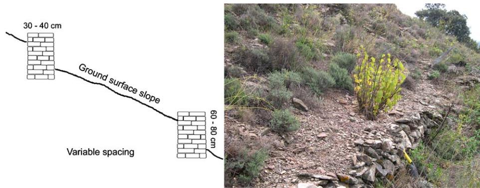
Fig. 2. Example of stone walls that composed the terracing system in the Priorat region in the past.
