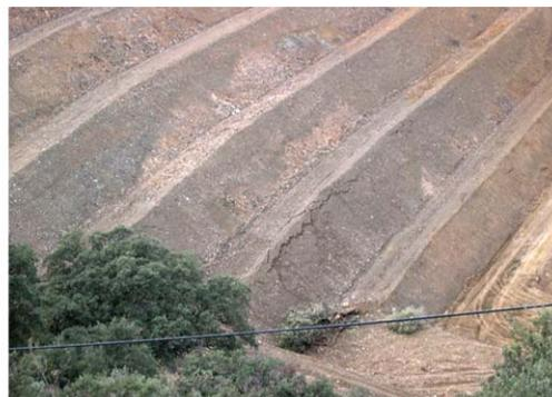
Fig. 3. Example of bench terraces constructed at present with heavy machinery in the Priorat region.
